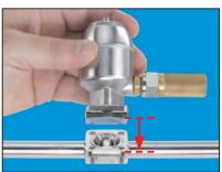
8. Place the actuator / bonnet with mounted diaphragm onto the valve body. Ensure that the valve body, diaphragm and compressor are in correct alignment.
